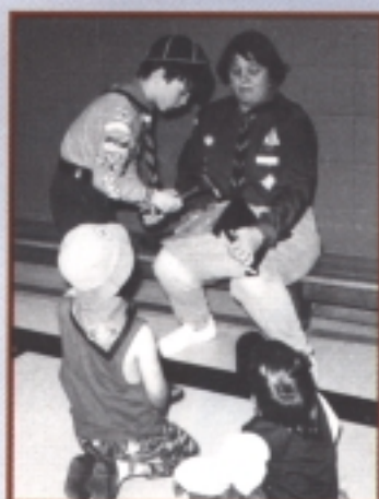
Raksha helps position a box while Cub Chris Arthur attaches tar paper to the roof. Bats need warm houses. The black paper absorbs heat and keeps out water.
